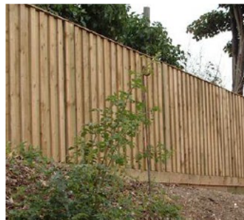
Img 28 - Timber acoustic fencing (Source: thewilddegrouop.co.uk)
