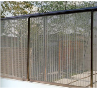
Img 25 - Steel mesh panel fencing (Source: Charles Elliot)
